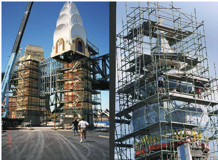
Early 1990's restoration work
